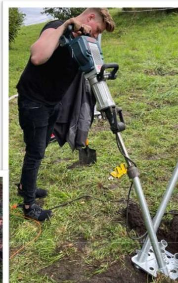
1. Remove any dirt and debris from the sections of the positioning module's pipes where the micro-piles will be driven into the ground, so that they can move smoothly during the installation process.
